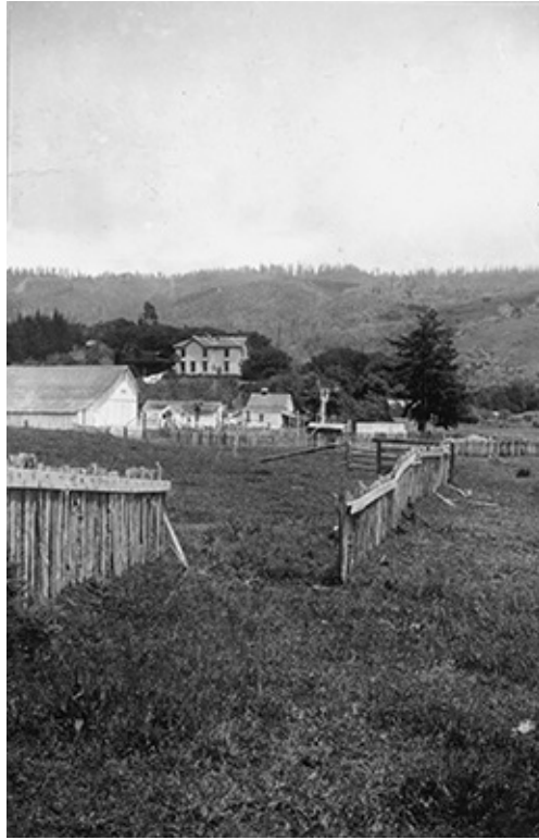
17. G. K. Gilbert's photograph of a fence offset in the San Francisco earthquake of 1906. The fence receding into the distance was displaced to the right relative to its continuation in the foreground on the left.
